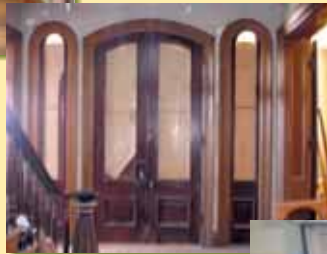
View of Interior Doors of Front Porch
